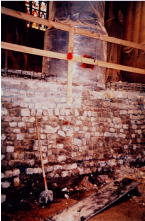
Figure 11: Chain wall between columns
